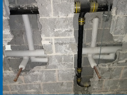
Continuing Insulation of Plumbing Lines in Building 2010
