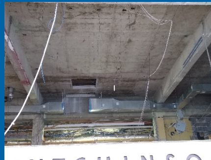
Roof Cut for New RTU and Installation of New Duct in Entry
