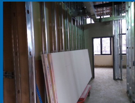
Installation of Drywall and Frames in Drywall at New Offices
