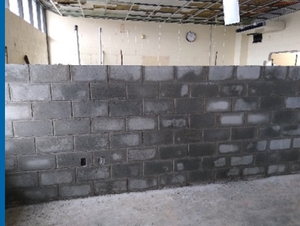
Construction of New CMU Walls in Building 2010 & 2020
