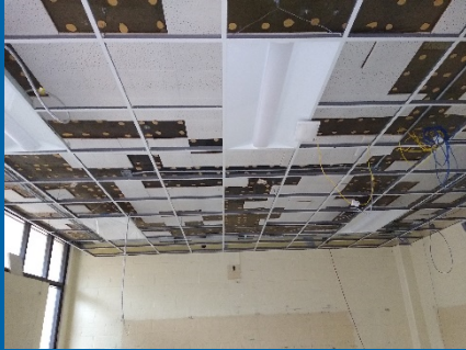
Installation of Lights in Building 2010 Classrooms
